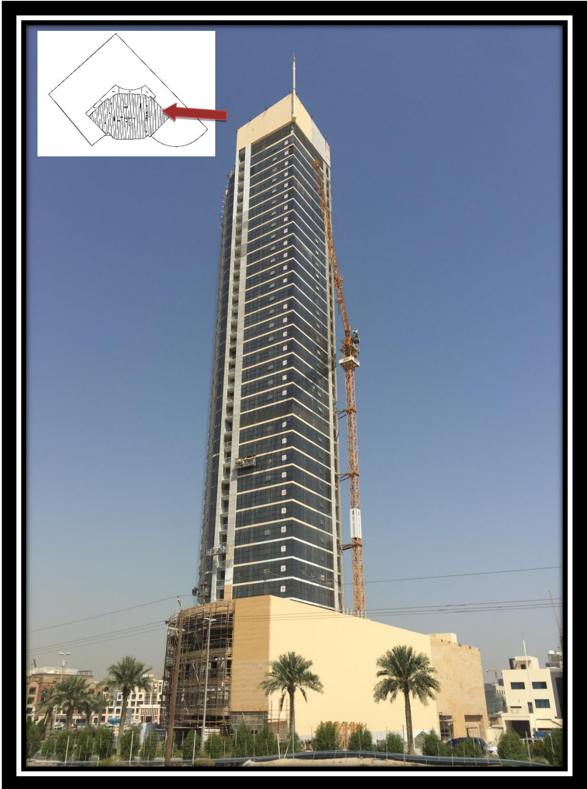
External Façade works- High Mast Installed
