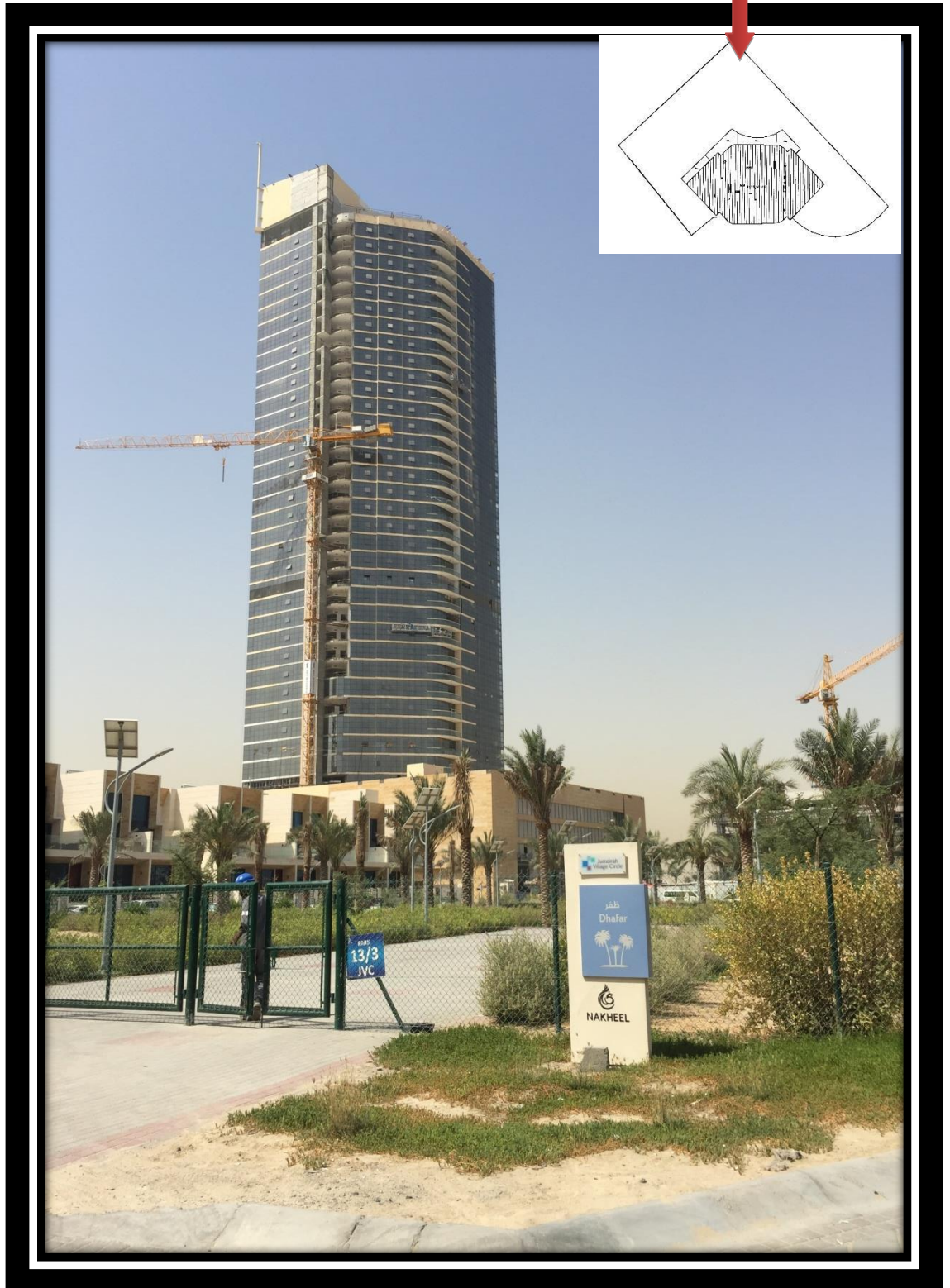
External Teak wood Stone cladding to podiums in progress.
