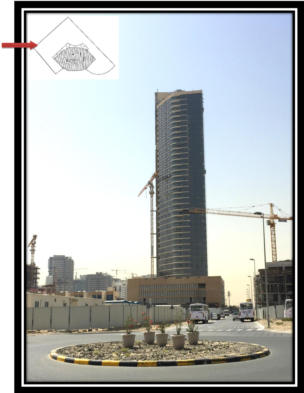
External Façade works
