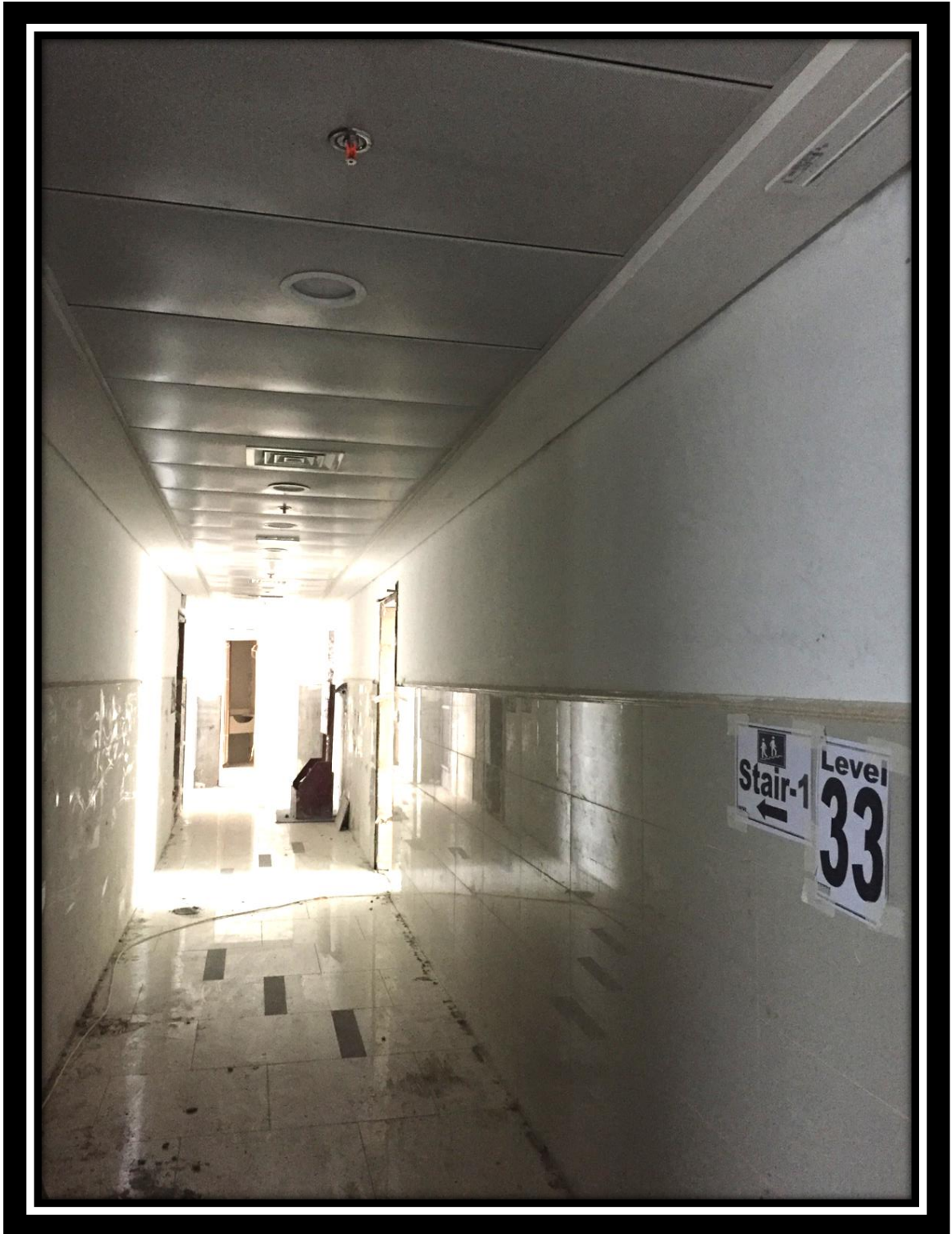
L-33 Corridor Finishes and Flase ceiling Closed
