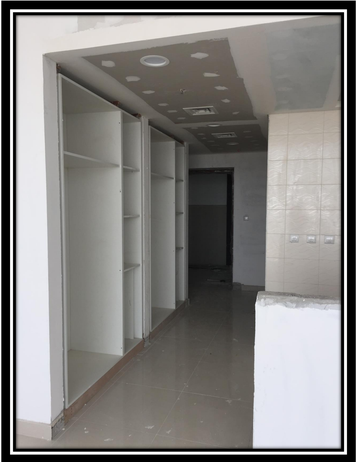
L-30 Light fittings, grills, ward robes and switches installed
