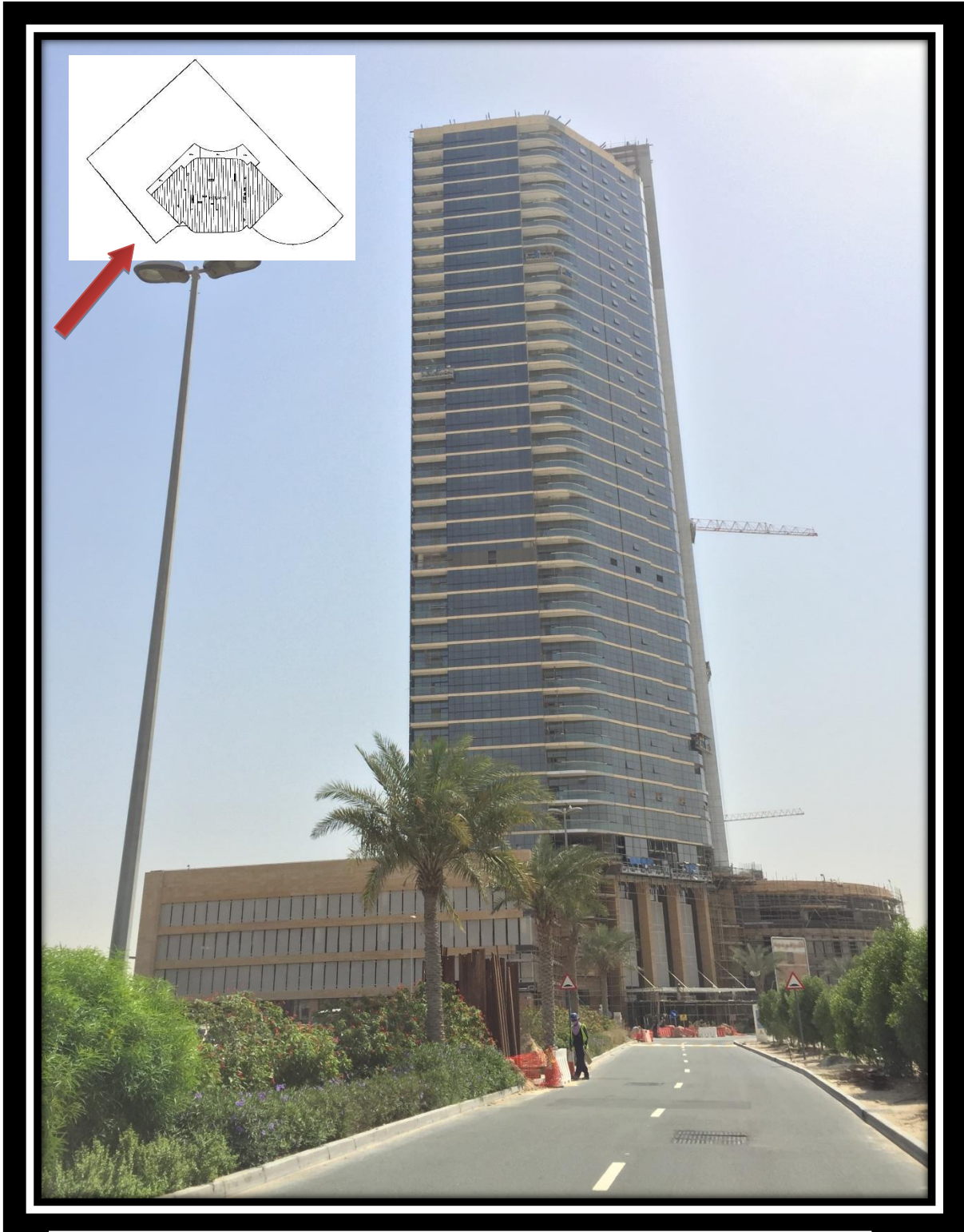
External Façade Completed
