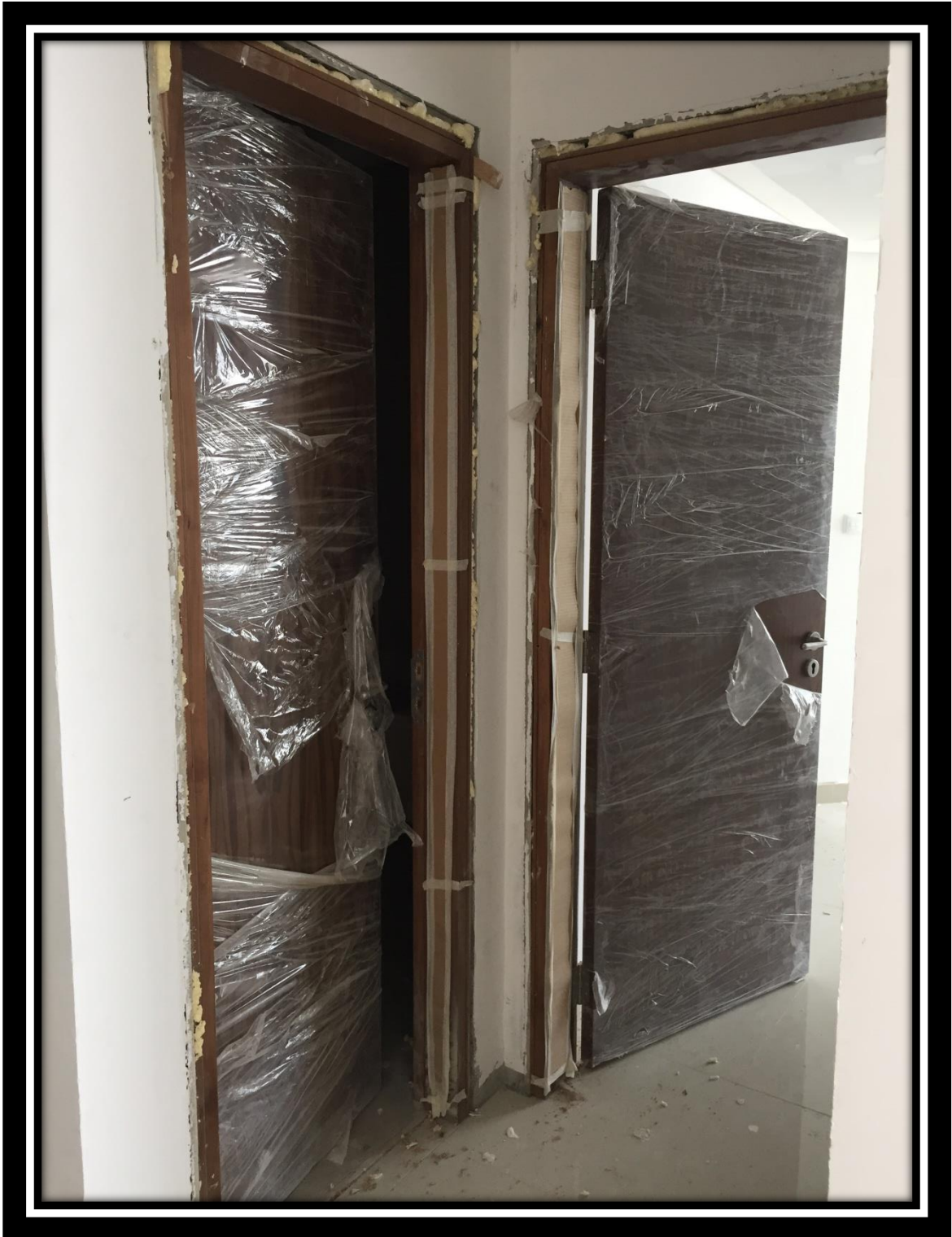
L-33 Door shutters installed
