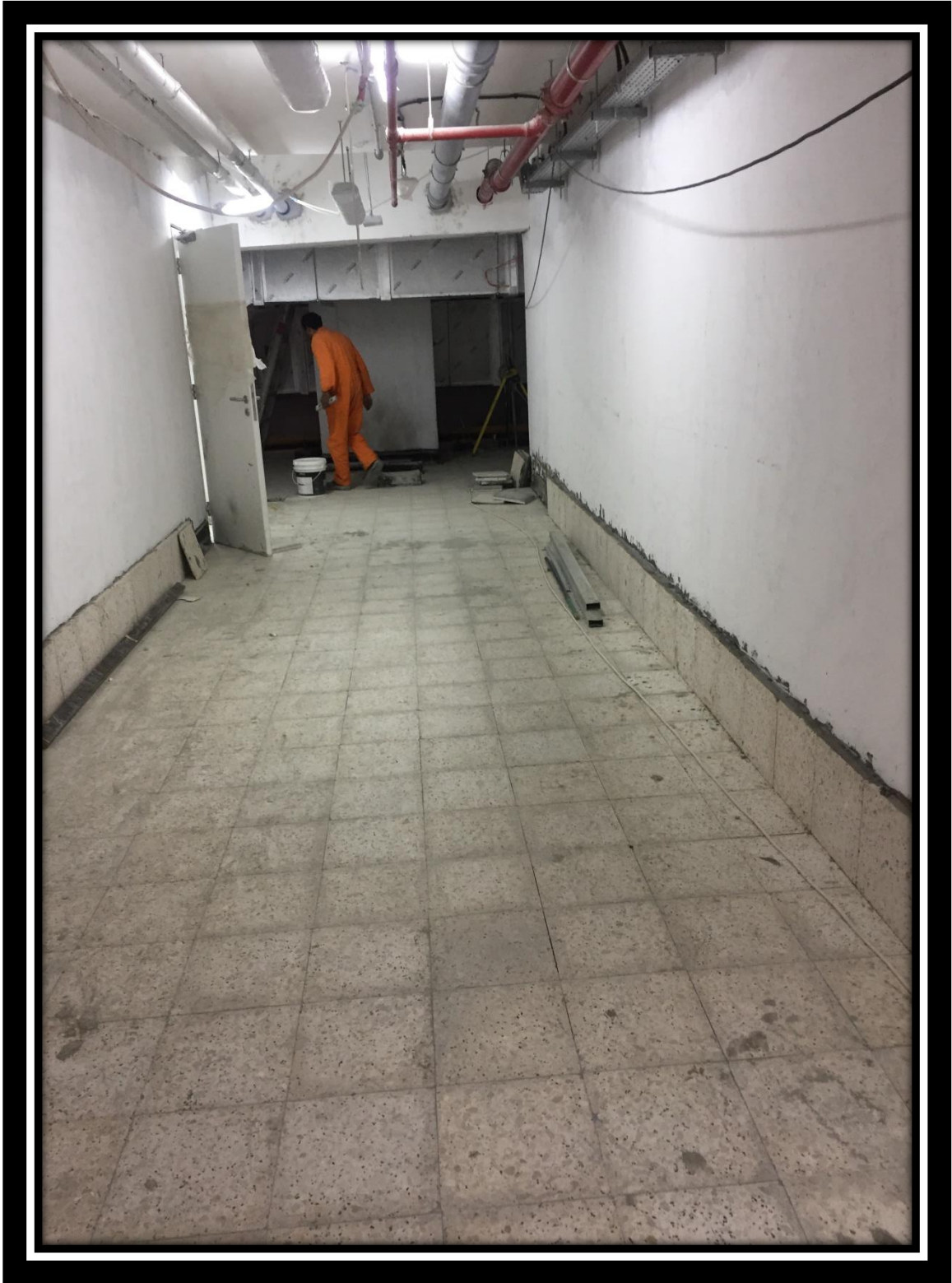
L-37 Mechanical floor Corridor finishes
